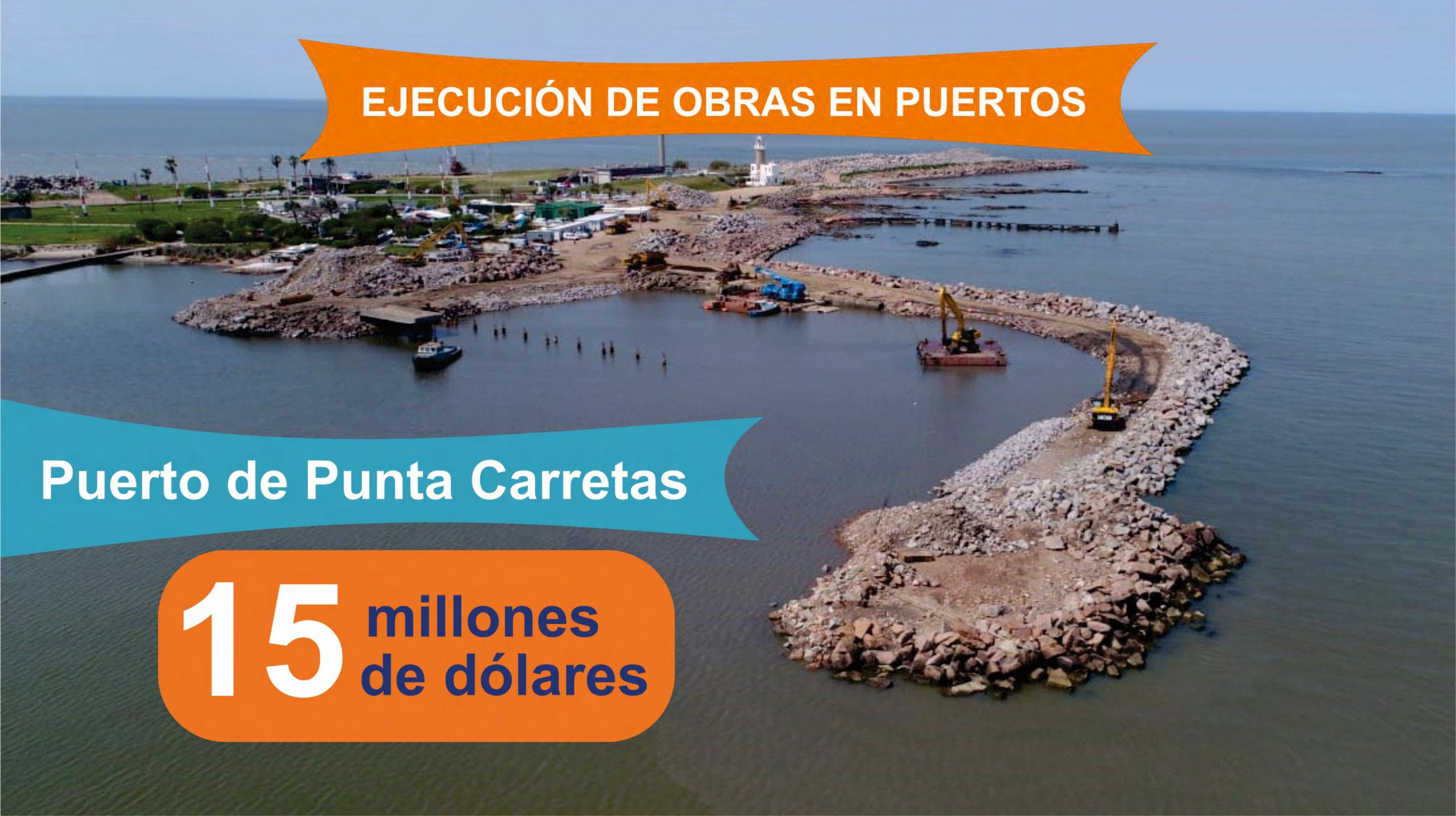
An aerial photograph showing a large-scale construction project for a port. A long, curved breakwater made of grey rocks extends from the shore into the sea. Several yellow excavators are positioned on the breakwater and in the water. In the background, a white lighthouse stands on a small island. The sky is clear and blue, and the water is a calm, greyish-blue.
